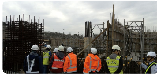
Safety patrol inspection operation
