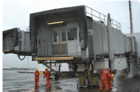
Bridge tying work
