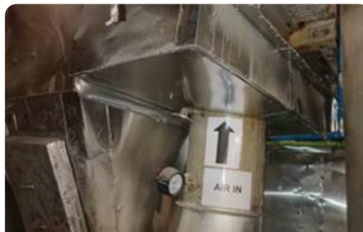
Replacement of Heat Exchangers
