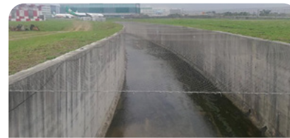
Set up bird nets over ditches
