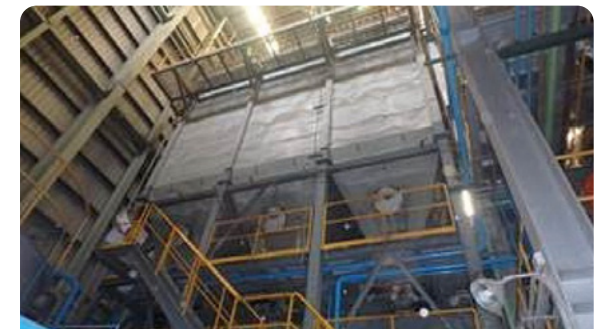
Inspection and repairs of Baghouse funnels
